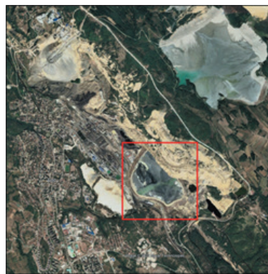
Figure 1. Satellite image of the location of the flotation tailings "RTH".
